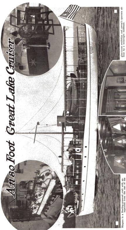
Sterling motors, and a 1 k.w., Fay & Bowen lighttion to crew's quarters is had forward, but the ing outfit as auxiliary equipment. Communica-The owner's quarters consist of two large, douowner's quarters aft are cut off by a bulkhead.
